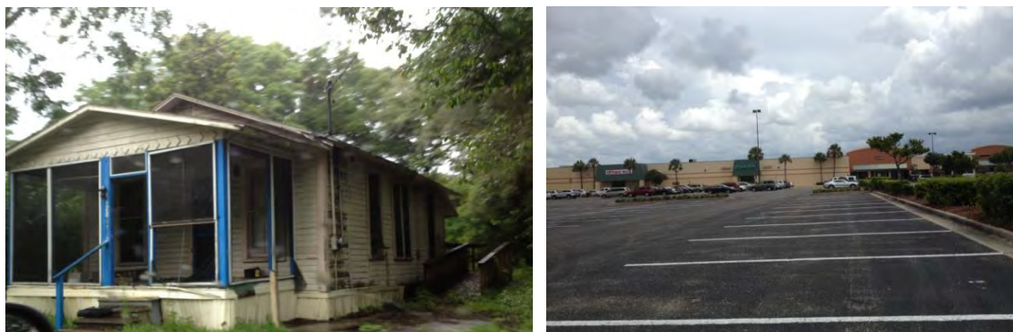
Figure 14: I-75 isolation has plagued West Ocala homes (left), spurring a need for streamlined downtown access. A typical sprawling development along Southwest College Road is pictured above on the right.
