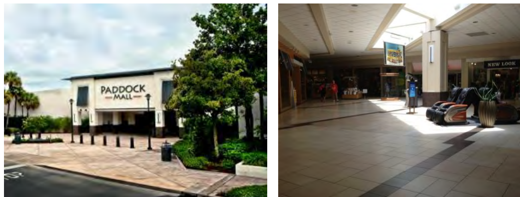
Figure 17: Paddock Mall features 554,000 sf of retail in Ocala, Florida, and is the closest regional center to the downtown site. (Image Source: (Left) simon.com)
